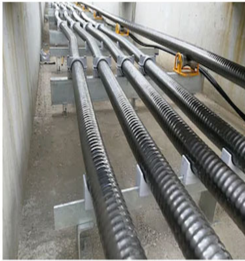
Cable Trench - With Pipe
